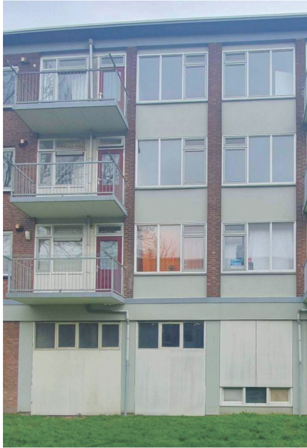
Figure 10a: Current courtyard. Before and after
