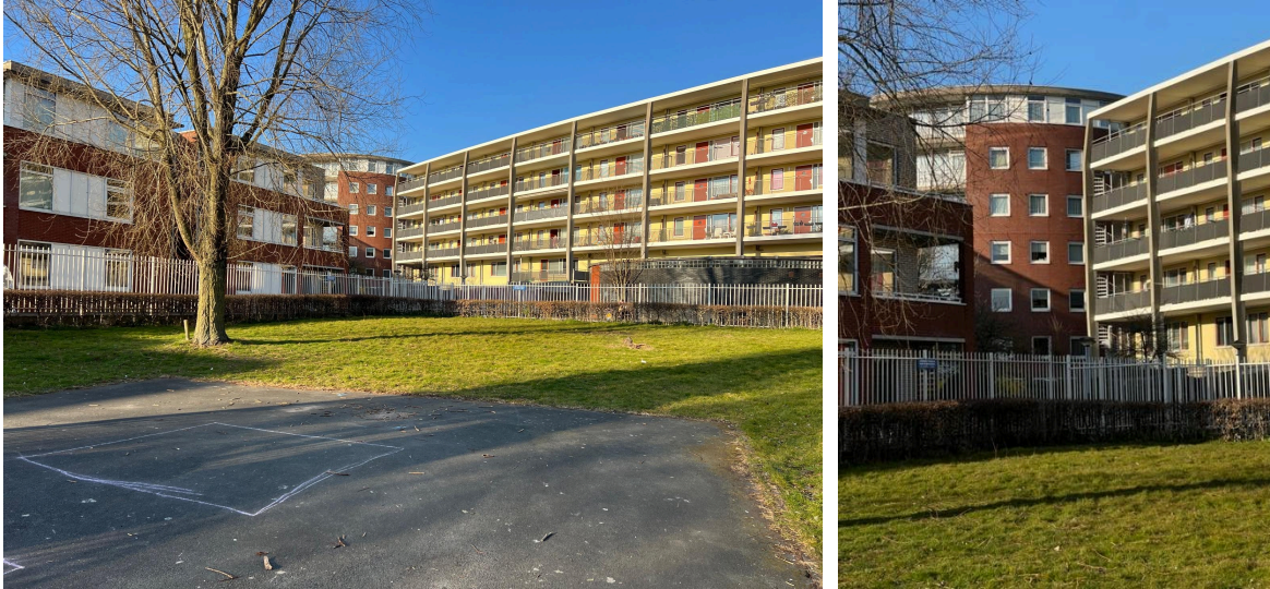
Figure 12: The fence between the Kamerrade and the park
